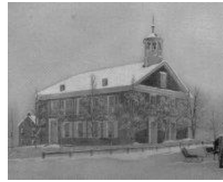
2705 West Canal Road, Dover, PA
